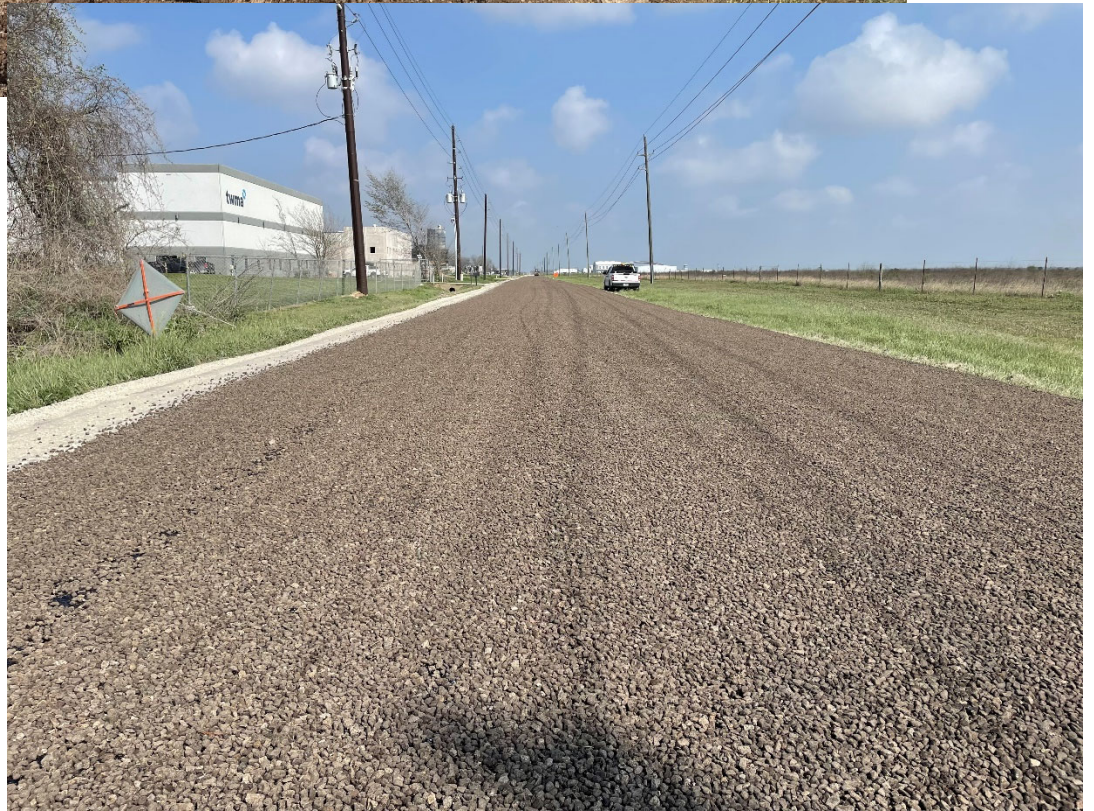
Above: WCRB operators stabilize road subgrade in advance of a seal coat project on Cardiff Road.
